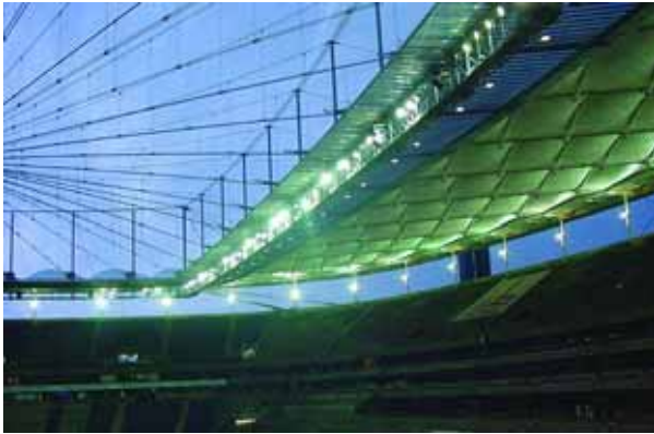
indirect illumination of the tribunes Commerzbank Arena, Frankfurt/M., Germany
