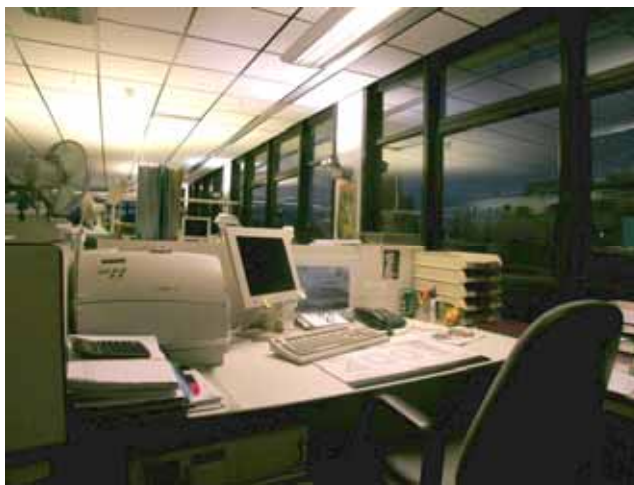
Fig 4. Direct-indirect suspended luminaire. Allow usage of 1.20 or 1.50m fluorescent tube. But work place cannot move if luminaire position is fixed. Leads to the lowest electrical consumption: 6W/m 2 . In open plan office. Could use 2x54 W fluorescent tubes for two people.
