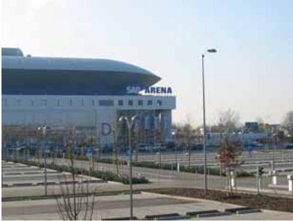
Outdoor Lighting SAP Arena Mannheim Germany
