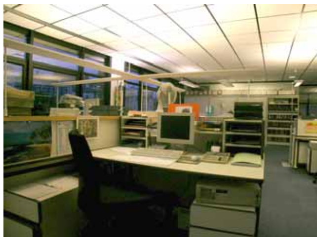
Fig 5. Indirect luminaire integrated to the furniture. Judged as very comfortable, the ceiling luminances are moderate, but the general feeling tends to have a work plane looking darker than the rest of the room. Requires about 2x35 W fluorescent tubes per work place.
